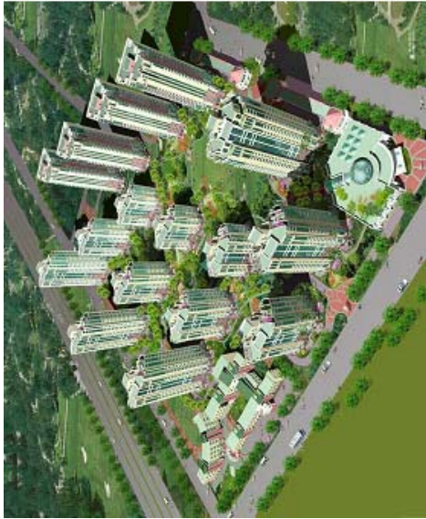
Figure 8 Beijing Star Garden - a high-rise residential development
