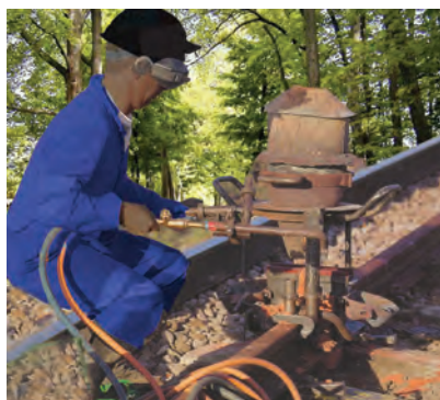
Figure 3.11 Thermit process for joining railway tracks
