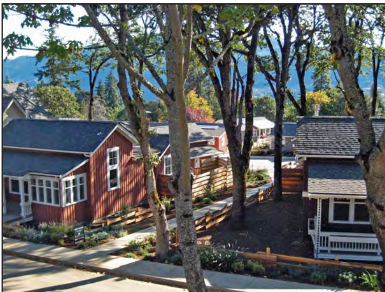
Live-work homes, Wyers End, White Salmon, WA. (Photo courtesy of Ross Chapin Architects.)
