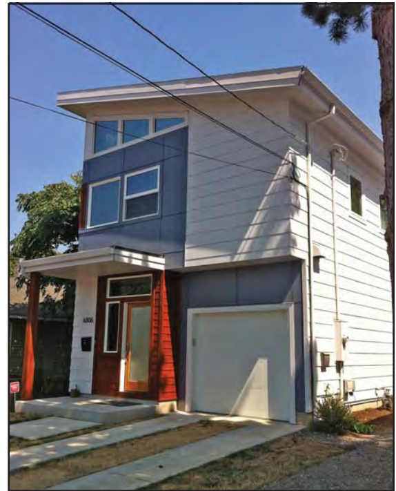
Street-facing main dwelling, Woodstock Gardens, Portland, OR (Photo courtesy of Eli Spevak.)
