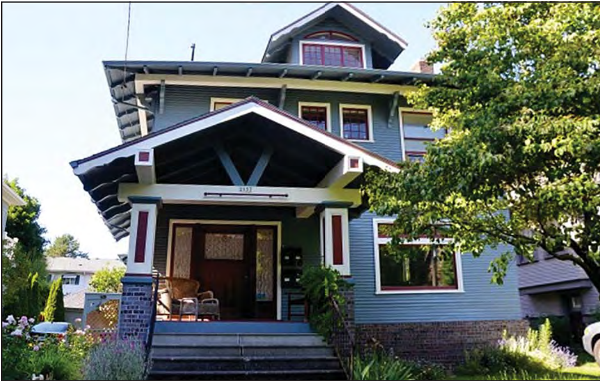
This four-plex still looks like a single-unit home from the street. (Photo courtesy of Michael Anderson, Bike Portland.)
