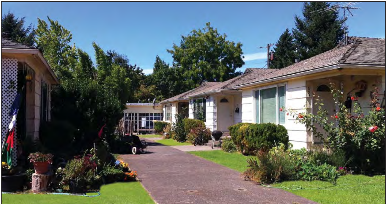
The Catterlin Cottages in Salem, OR, are six detached one-story homes, each approximately 38'x24', fronting onto a central courtyard. (Photo by Eli Spevak.)
