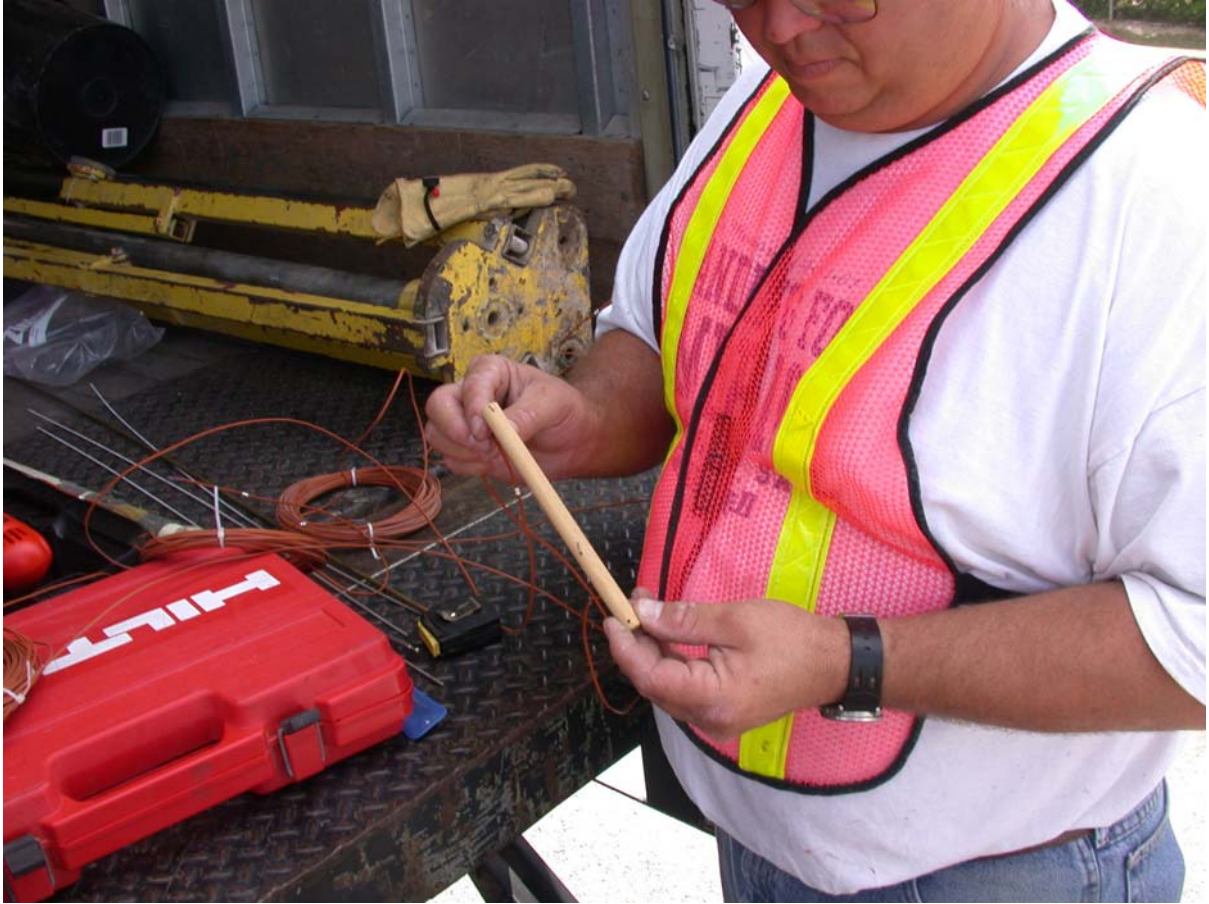
Figure B12. Wooden Rod Used to Install Thermocouple Wires.
