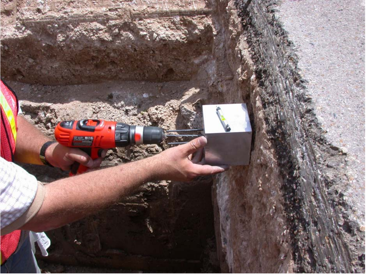
Figure B8. Drilling Holes for Installing TDR Probes.
