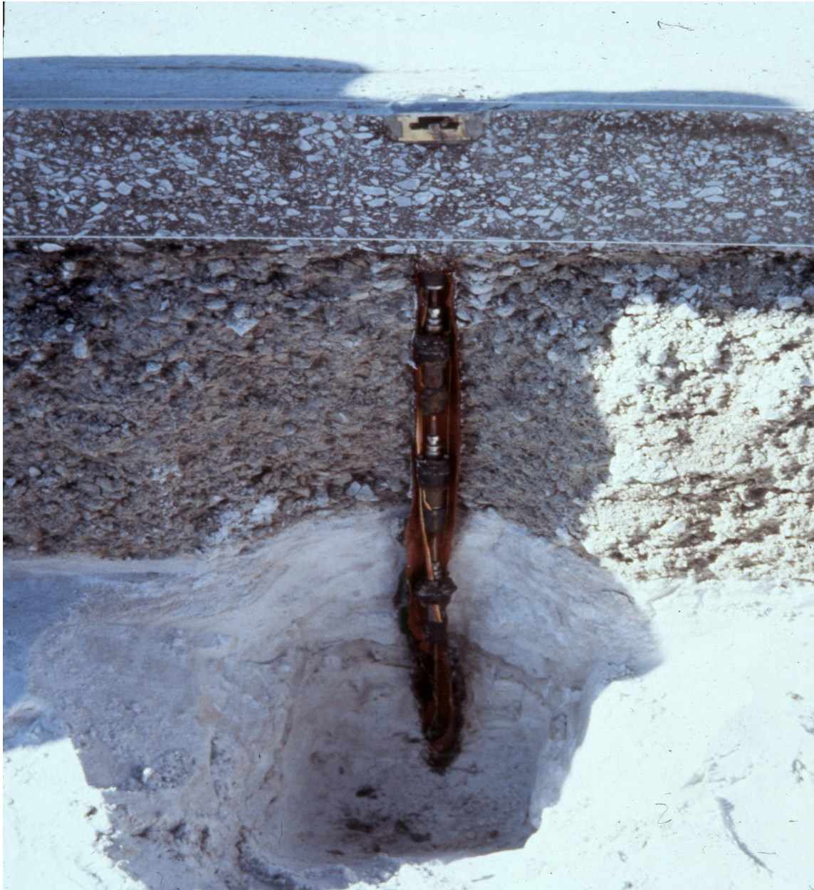
Figure 2.4. Picture of Trenched Pavement Showing MDD Installed within Test Section.
