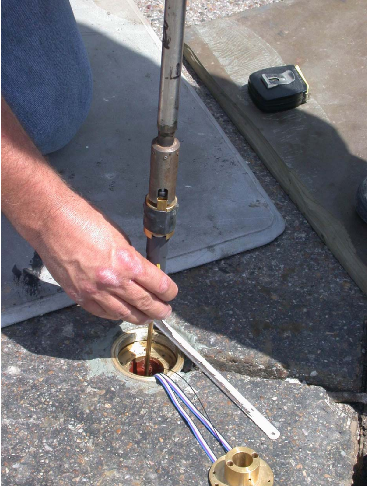
Figure B13. Installation of MDD LVDT Module.
