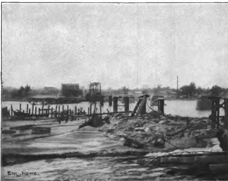
B. KANSAS CITY SOUTHERN RAILROAD BRIDGE, KANSAS CITY, AFTER THE FLOOD.
