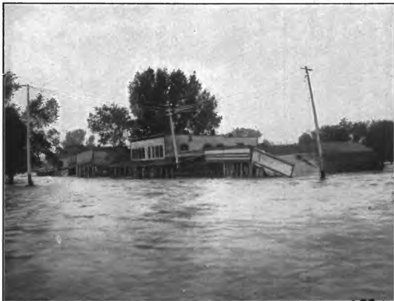
A. BRIDGE STREET, NORTH LAWRENCE, KANS., DURING THE FLOOD.
