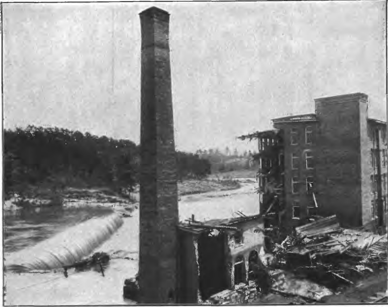
A. VIEW OF DAMAGED PORTION OF PACOLET MILL, NO. 3.
