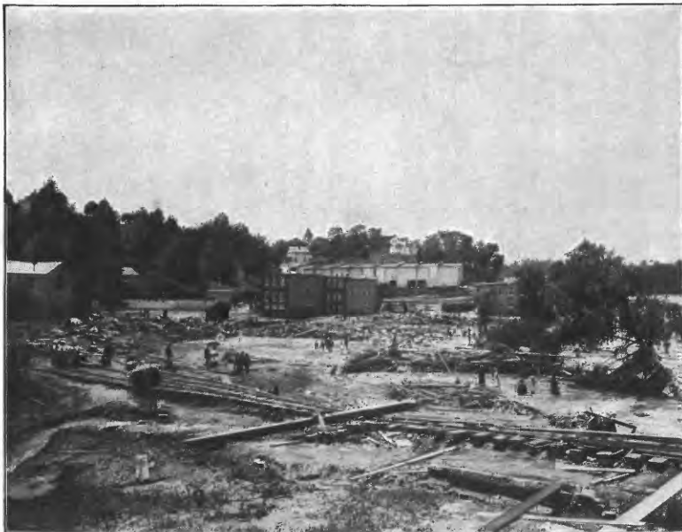
B. VIEW OF WRECKAGE OF PACOLET MILLS, NOS. 2 AND 3.
