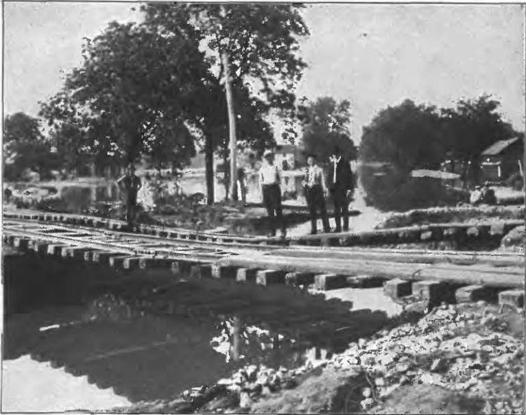
A. UNDERMINED SECTION OF RAILROAD NEAR LAWRENCE, KANS.
