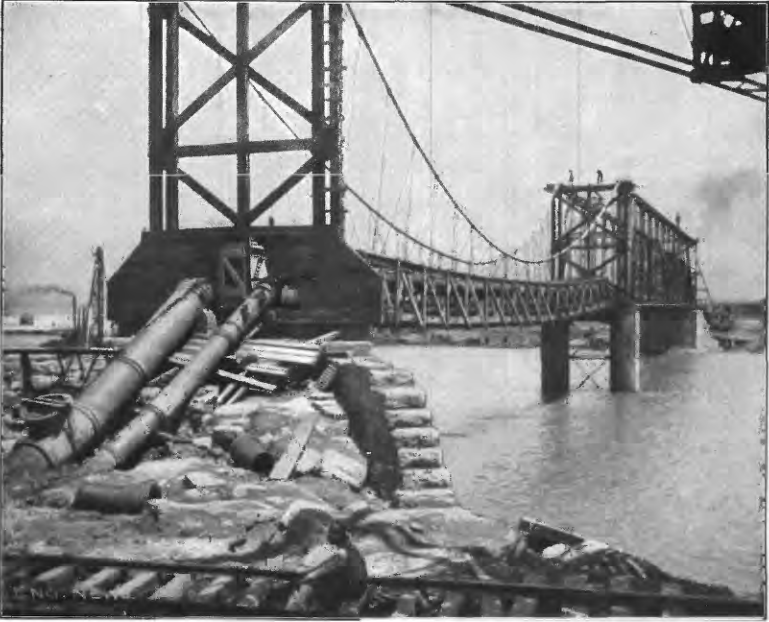
A. VIEW OF "FLOW-LINE" BRIDGE, REPAIRED WITH SUSPENSION SPAN.
