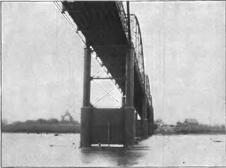
A. BRIDGE AT LAWRENCE, KANS.
