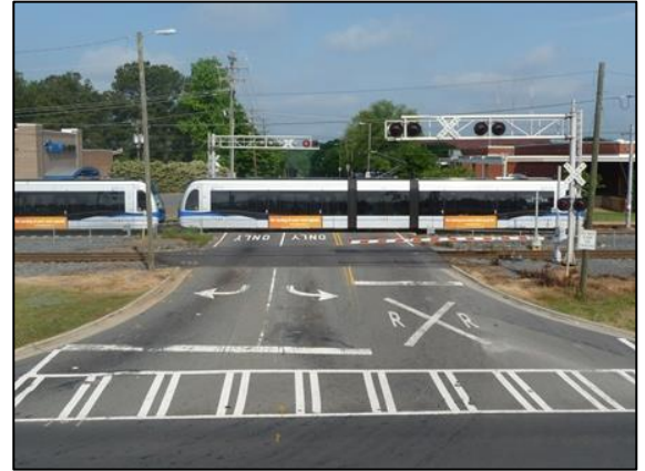
CATS light rail and NS freight tracks at-grade crossing at Hebron Street
