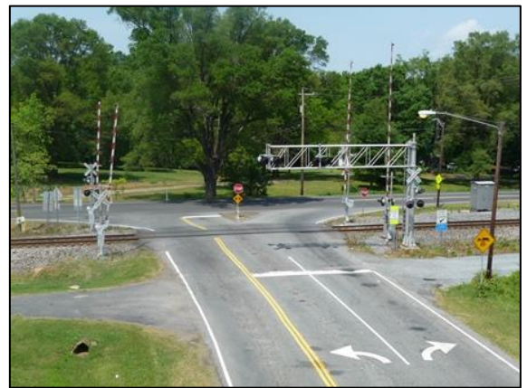
Before: The NCR/ Newell Hickory Grove Road crossing to be closed as part of NCDOT's Piedmont Improvement Program in 2016.
