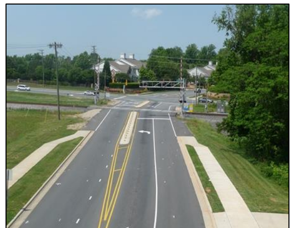
Intersection improvements at NCR/McLean Road rail crossing near Old Concord Road.
