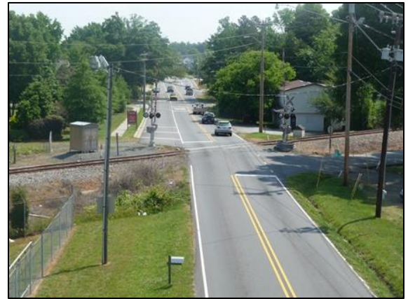
Current NS freight track (future LYNX Red Line commuter rail line) at-grade crossing at Nevin Rd.
