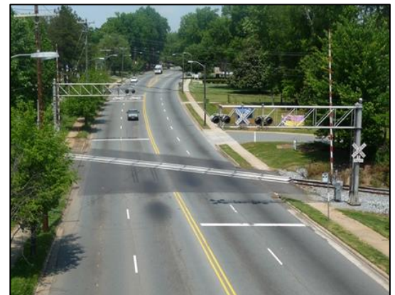
ACWR crossing at Eastway Drive
