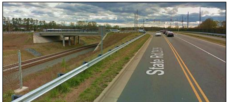
Grier Road overpass over NCR (view from Old Concord Road)
