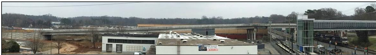
Sugar Creek Road grade separation over NCR and LYNX Blue Line light rail
