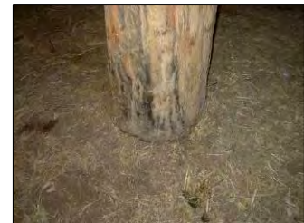
Rotting post footings need to be replaced.
