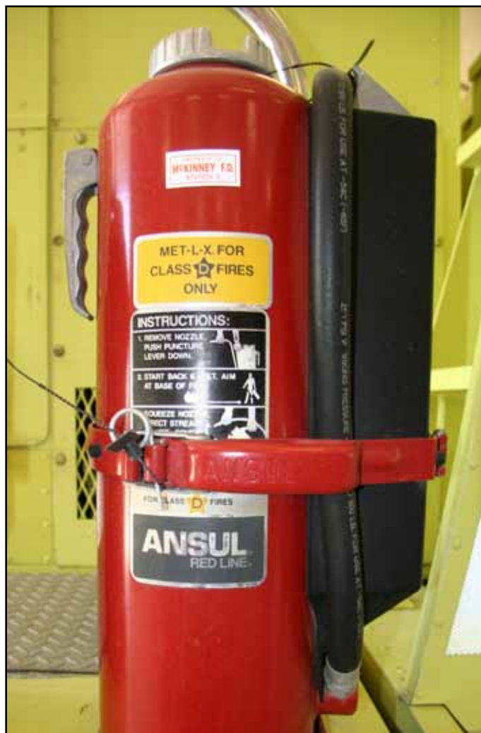
Figure 4.46 Class D extinguishers are designed for water-reactive metal fires.
