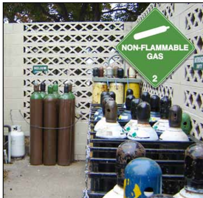
Figure 4.17 Inert gases are nonreactive, but they can cause asphyxiation by displacing the oxygen in confined spaces.
