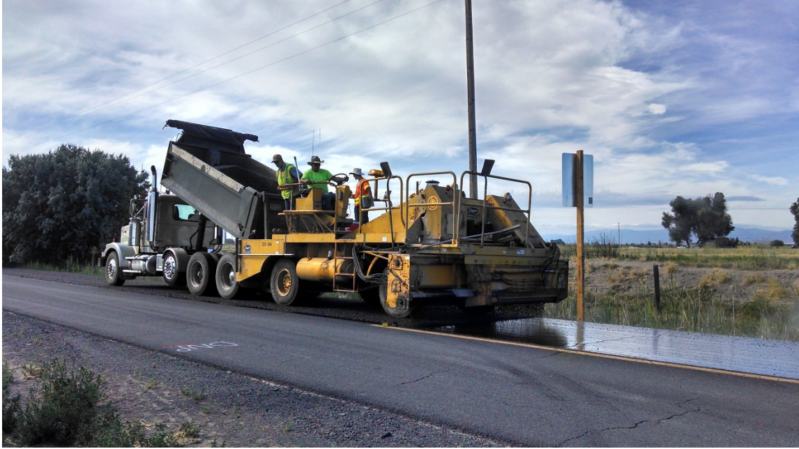
Figure 4.4: Aggregate Laydown Operation (Photo credit: Paul Ledtje)
