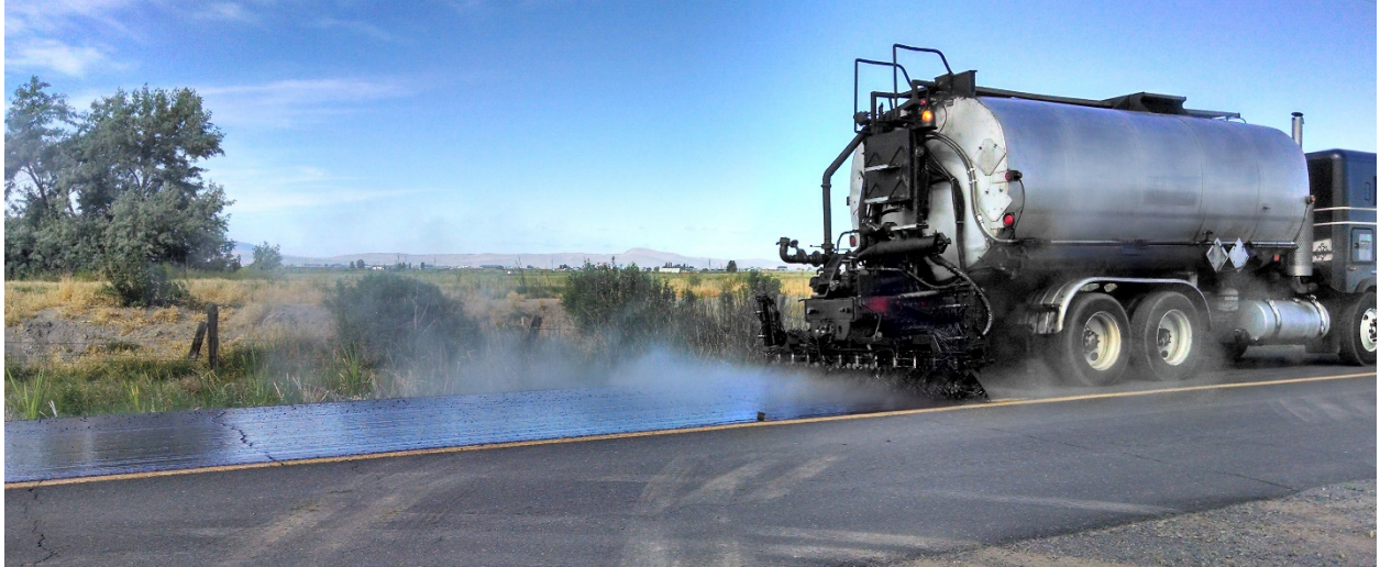
Figure 4.2: Chip Seal Distributor Spray Bar (Photo credit: Paul Ledtje)
