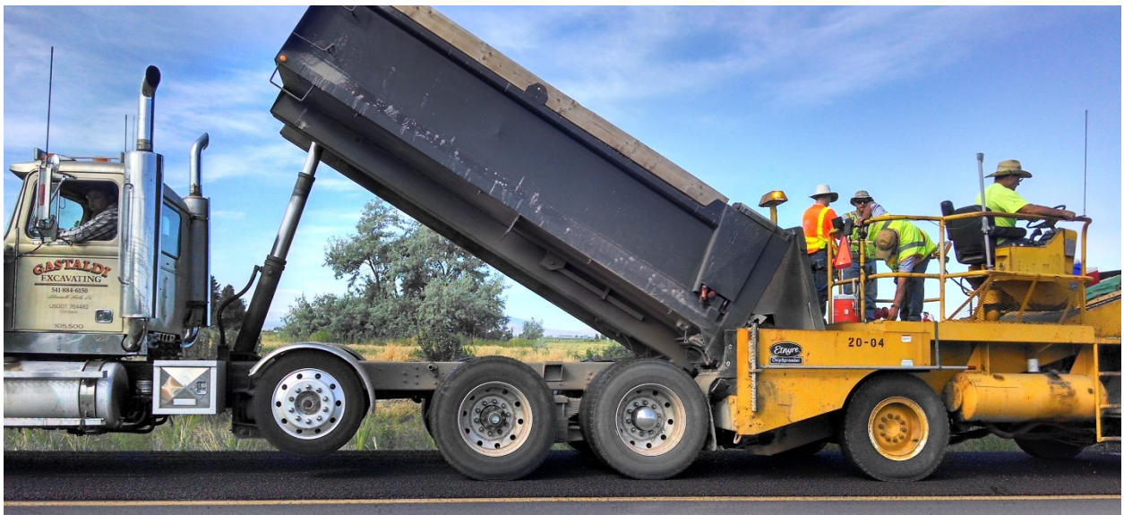
Figure 4.3: Haul Truck Loading Chip Spreader (Photo credit: Paul Ledtje)
