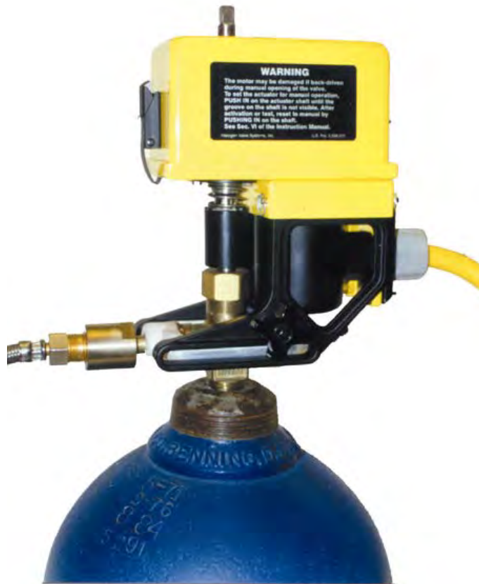
Automatic Actuator - 150 Lb Cylinder
