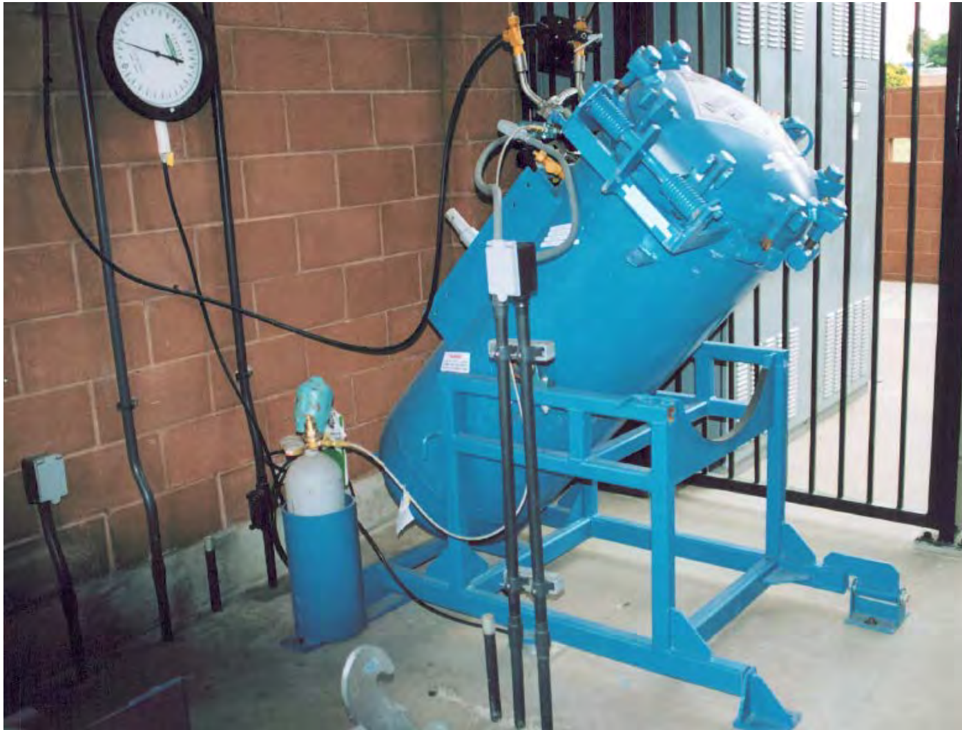
Typical 150 Lb Cylinder Containment System
