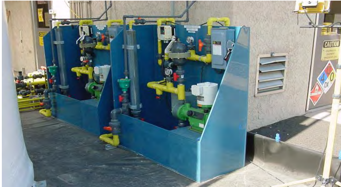
Typical Sodium Hypochlorite Dosing Station
