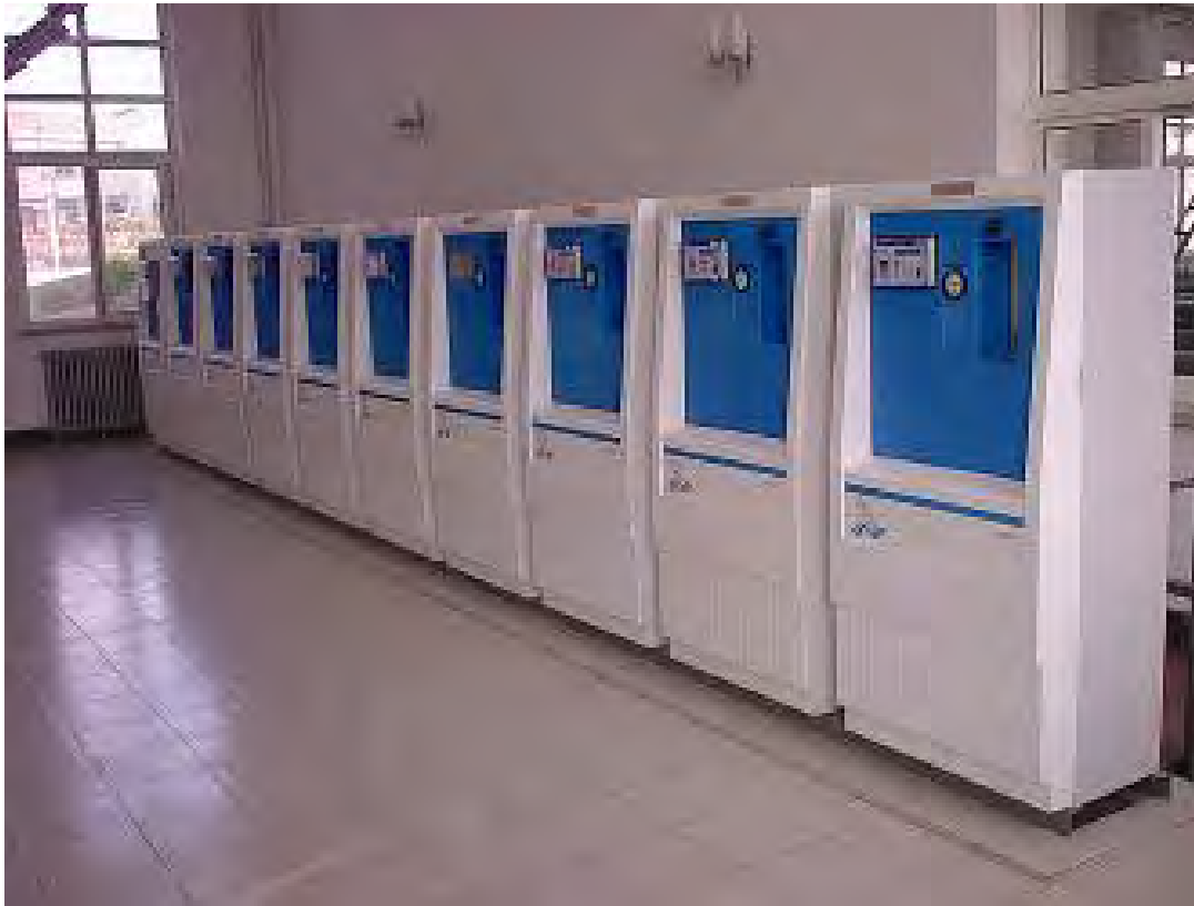
Typical Chlorine Gas Feed System
