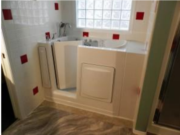
Escape Plus Walk-in tub installed with deck extension and custom tile.
