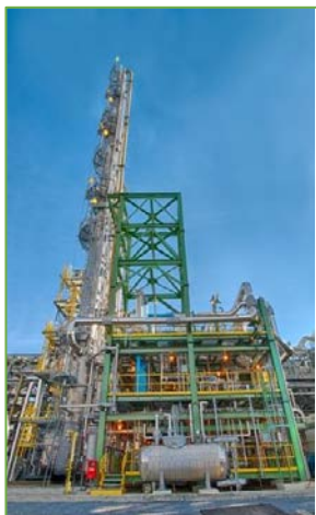
1.5 MWe Solvent Pilot (Linde and BASF)
