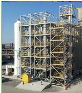
0.7 MWe Solvent System (Univ. of KY – CCSI - Hitachi)
