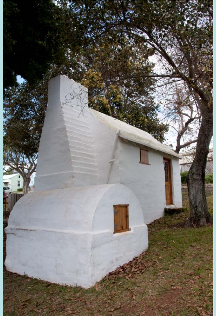
In this historical home, the door of cistern is used to retrieve water.
