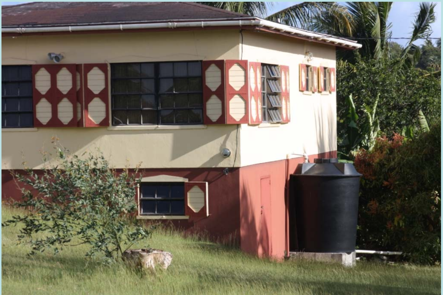
This rain barrel is used simultaneously with water piped into the house.
