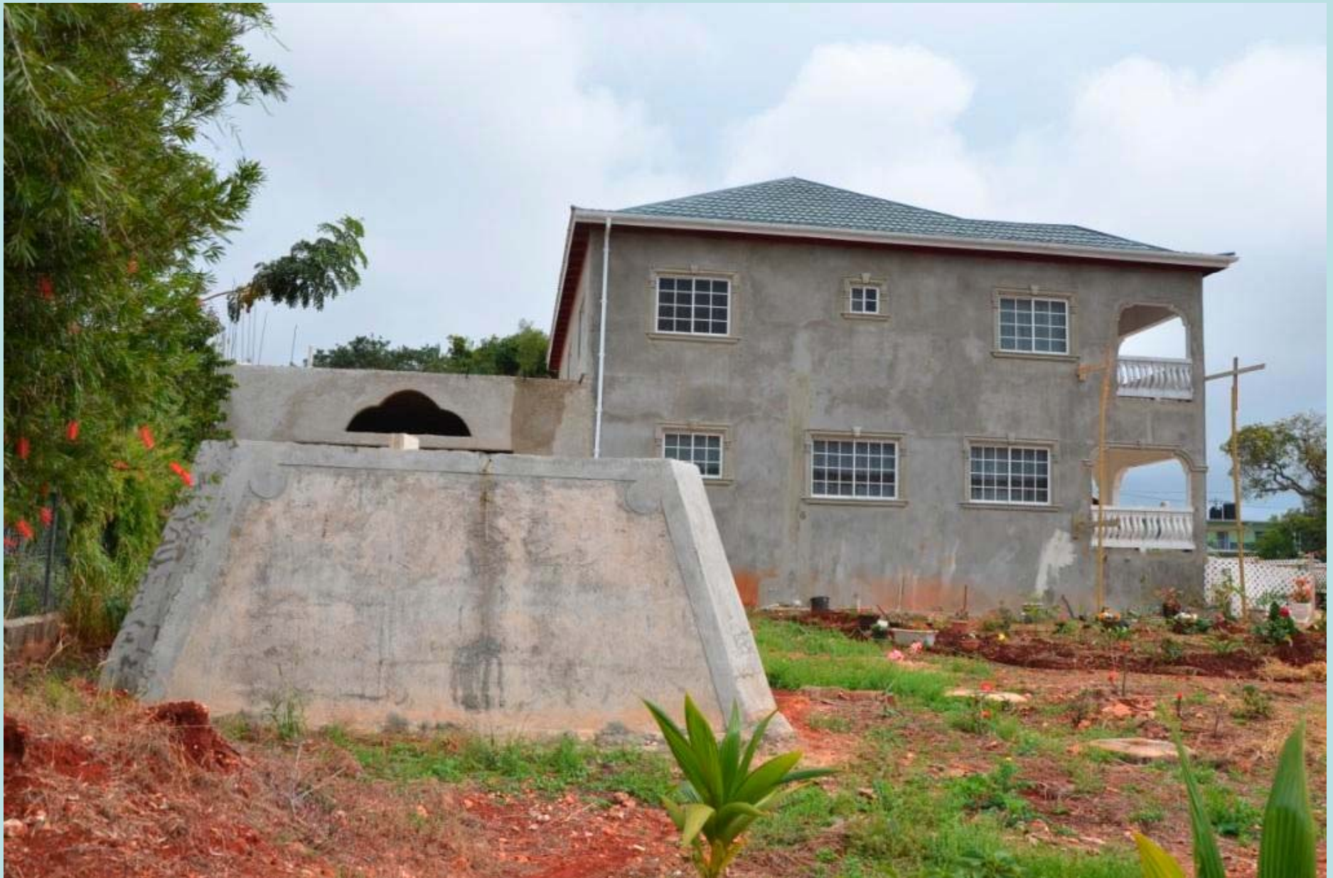
A new house and a new cistern. This cistern is much larger than the one in the previous slides. The method of collecting water has not changed. South Field, Jamaica
