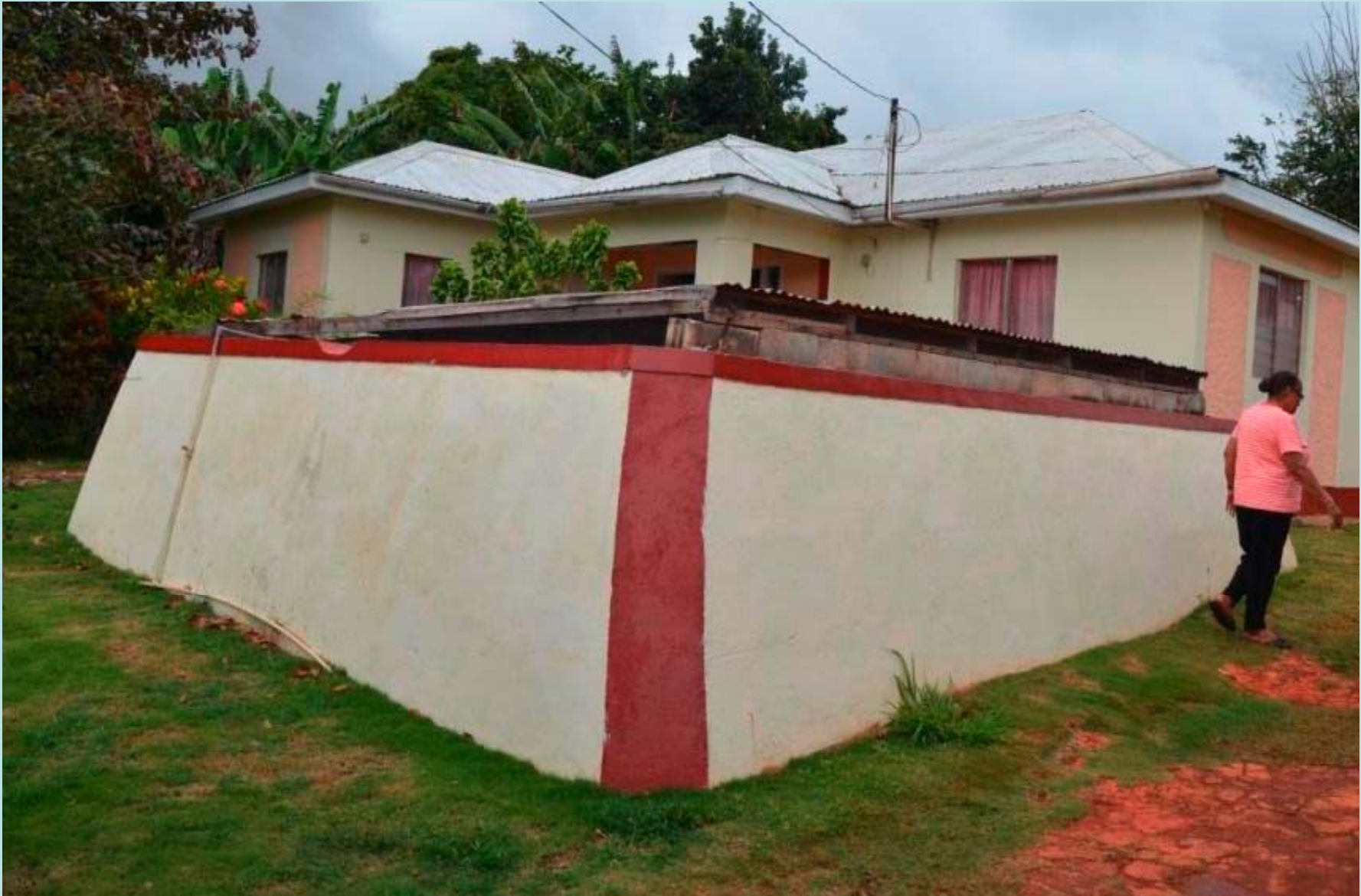
The above ground dimension of this cistern is 20' long, 18' wide, and 6' tall at its highest end. It is roof fed. Southfield, Jamaica
