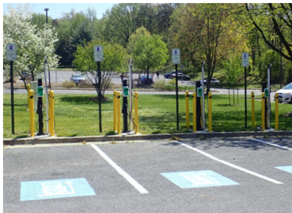
Four L2 chargers at the Schrom Hills Park offer public charging in East Greenbelt.
