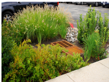
FIGURE 10.26 RAIN GARDEN IN PARKING LOT
