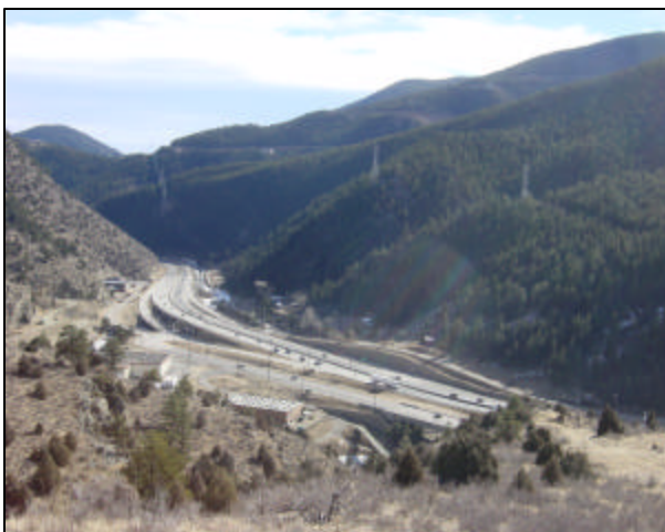
View to east above Hidden Valley Interchange
