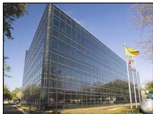
2400 Veterans office building in Kenner
