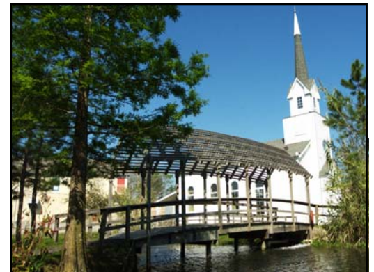
Church and covered bridge in Heritage Park, Rivertown
