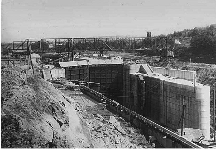
Figure 5. The same vicinity as in Figure 3, ten years later. The construction of Seattle's ship canal, today named after chief engineer Hiram M. Chittenden, linked Puget Sound (behind the photographer) to Lake Union (in the distance) and Lake Washington (over the horizon). The locks radically transformed Seattle's urban watersheds and in many ways brought an end to indigenous Seattle. The home of Hwelchteed, who was relocated to an Indian reservation across Puget Sound just before construction began, stood immediately to the right of this photo. Negative 2002.3.2022, Museum of History & Industry (MOHAI), Seattle.
