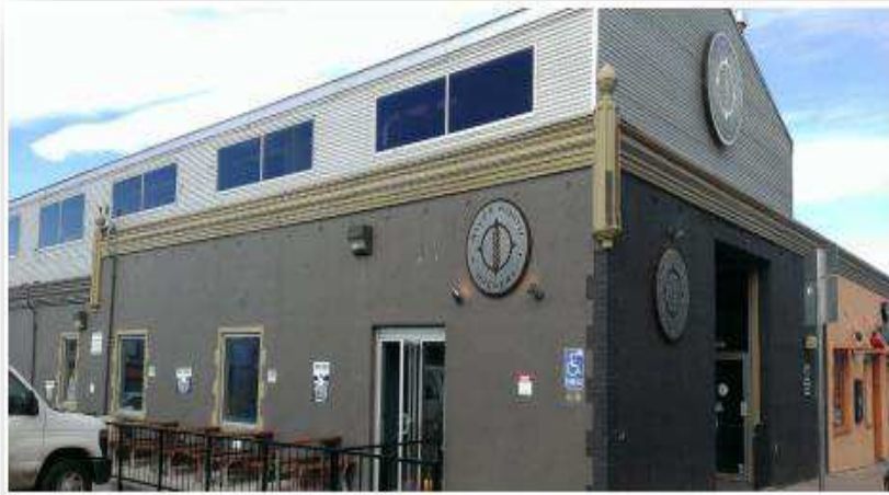
Examples of adaptive reuse of an industrial building in the (River North) RINO District of Denver.
