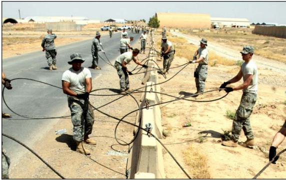
Figure 11.5. Constructing Security Barrier around Flightline.
