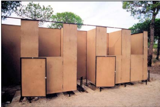
Figure 6.4. Straddle Trench Latrine with Partitions.
