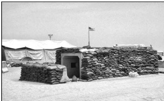
Figure 11.3. Improvised Bunker Using Concrete Culverts and Sandbags.
