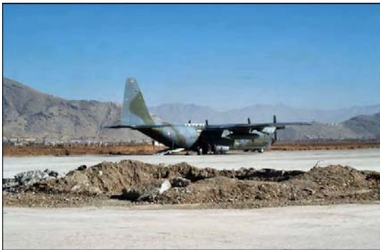
Figure 4.6. Crater with Upheaval.
