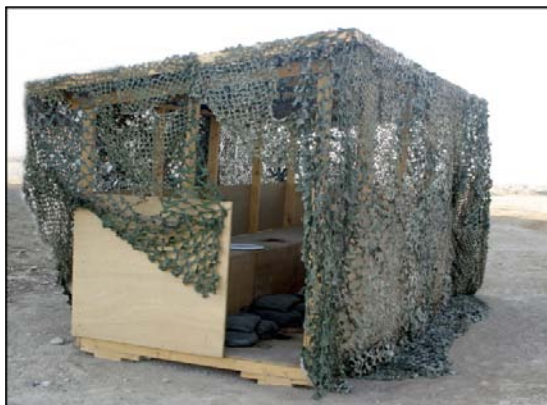
Figure 6.1. Field Expedient Latrine Often First Sanitation Facility.
