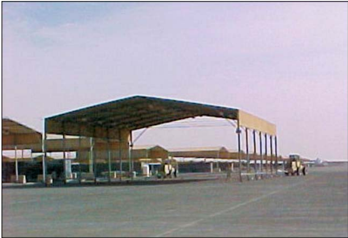
Figure 5.7. Engineers Relocate Aircraft Sunshades.
