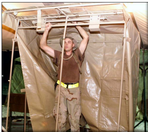
Figure 1.10. Assembling Field Showers at Operating Location.
