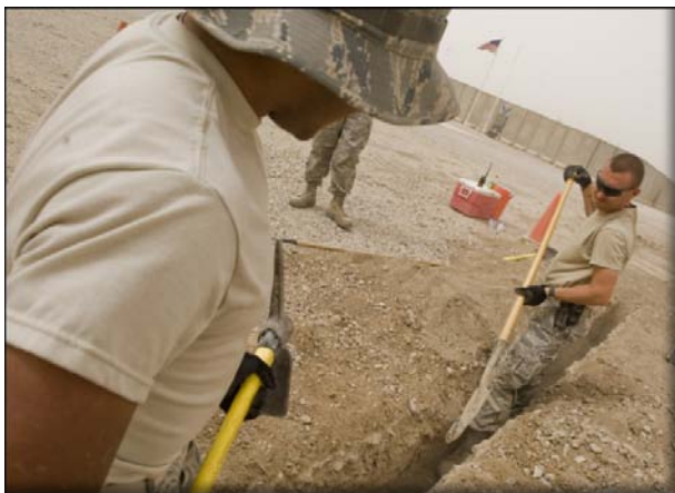
Figure 1.13. Digging Trench for Water Lines at Ali Base, Iraq (2008).
