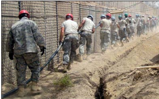
Figure 9.8. Burying Electrical Distribution Cable.
