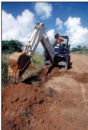
Figure 4.18 Creating Drainage Ditch to Reduce Road Erosion.
