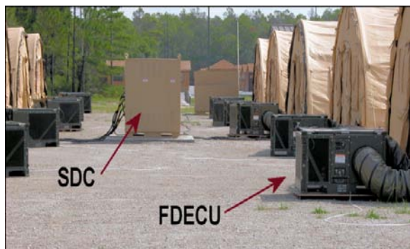
Figure 9.6. Typical SDC/Facility Configuration with FDECUs.
