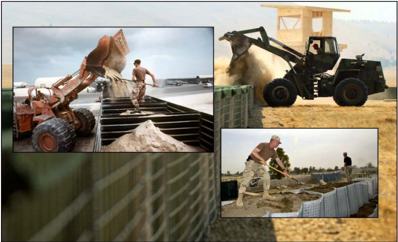
Figure 4.12. Expedient Revetments at Deployed Locations.
