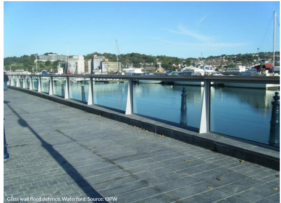
Glass wall flood defence, Waterford. Source: OPW
