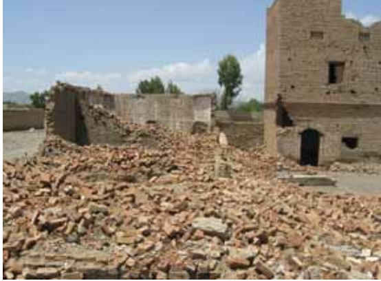
House destroyed by drone strike
