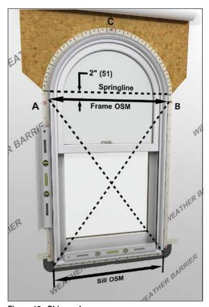
Figure 16: Shim and secure
