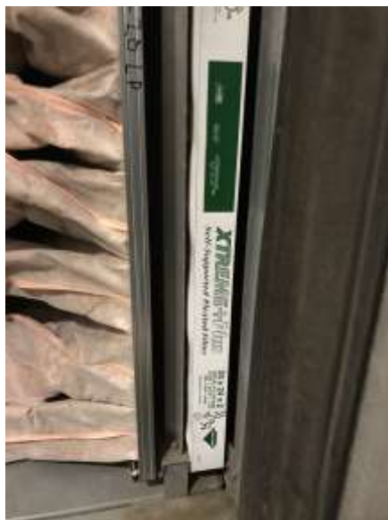
Figure 1: AHU-3 Pre and After Filters
