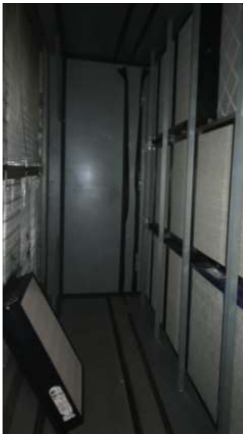
Figure 2: AHU-4 after filter blown out
