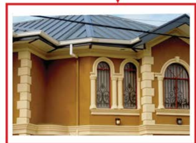
Quoins and engaged pilasters
