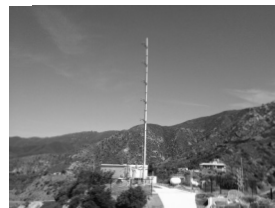
KDB Gibraltar Peak Tower Facility
