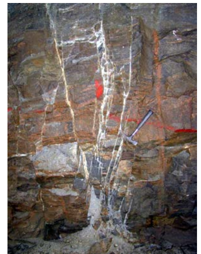
Figure 44: A small weakness zone with thin seams of swelling soil/clay
