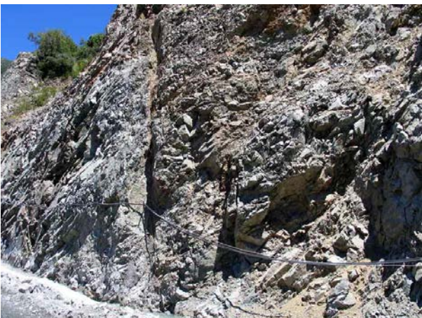
Figure 16: A filled joint/shear (singularity) intersecting a volume of jointed rocks.
