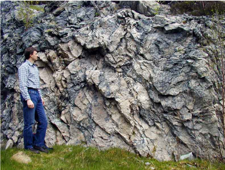
Figure 40: Irregular jointing. How to estimate RQD or block size correctly here?
