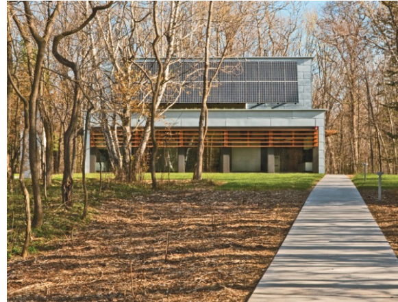
FIGURE 8. BAGLEY CLASSROOM, UNIVERSITY OF MINNESOTA DULUTH
