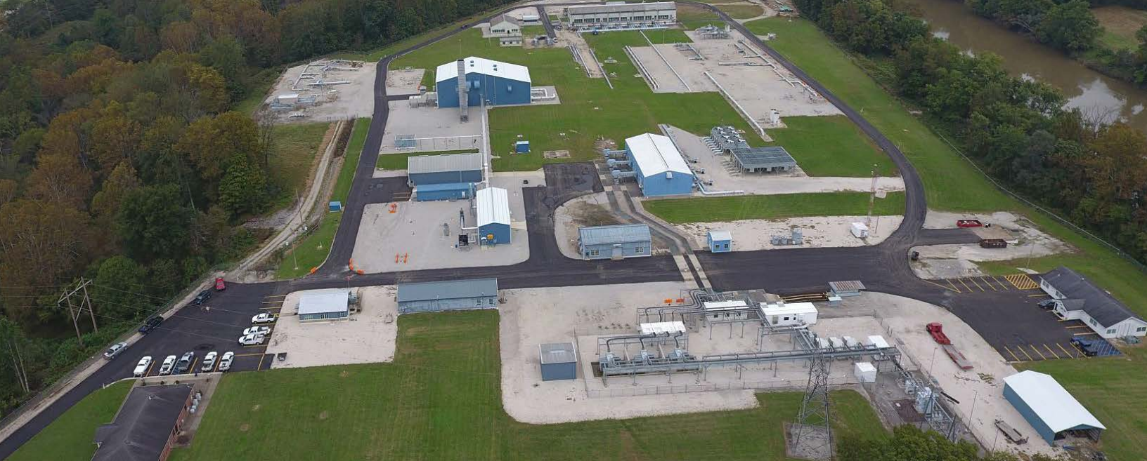
Compressor stations play an important role in transporting natural gas from the well to end users by sustaining the pressure and flow of natural gas. Note the pictured compressor station was not the one modeled in the study. Photo courtesy of Kinder Morgan
