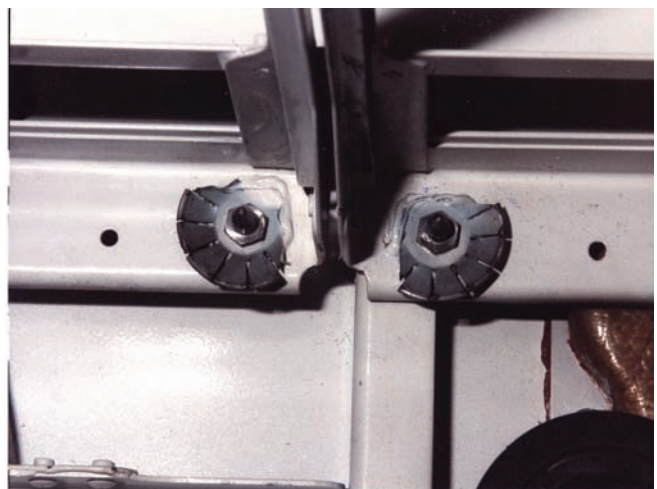
Figure 6-5. EMI Bonding Washers in Avionics Bay
