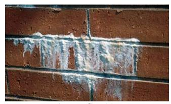
A severe case of lime staining
