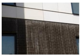
Staining from runoff over adjacent concrete components
