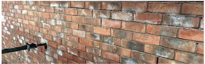
Efflorescence on brickwork under construction
