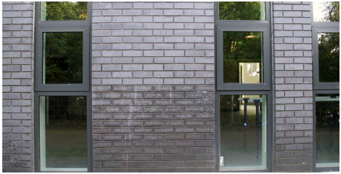
Picture framing likely due to saturation during construction
