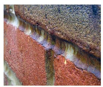
Iron staining visible on a mortar joint
