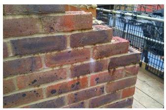
Staining on saturated brick work
