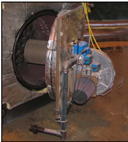
Figure B6-8. ClearFire-H burner
