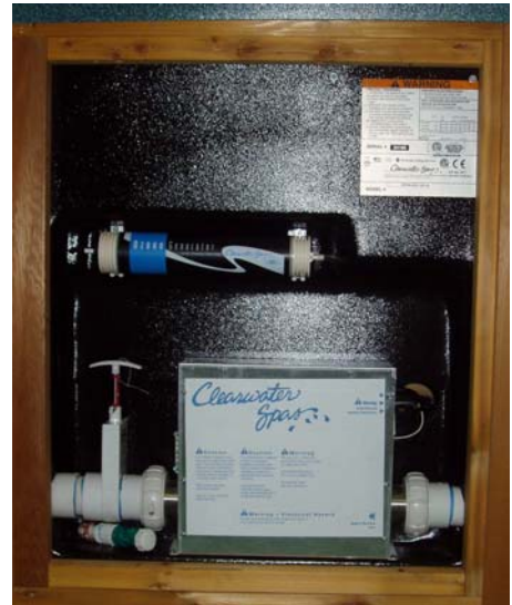
Figure 1-2 – Controller, Ozonator and Drain Valve
