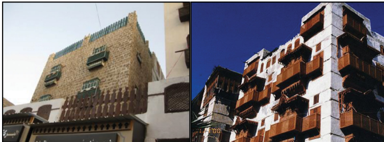
Figure 6: The materials that are used in the construction of Hejaz's buildings [7].
