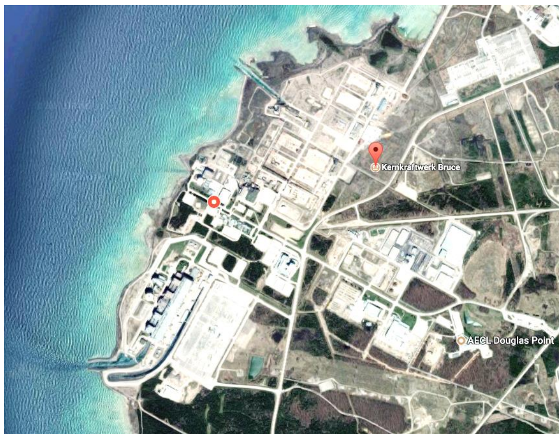
Figure 20: Imagery of a Nuclear Plant
