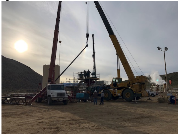
Figure 4: Installation of Vacuum-Insulated Tubing
