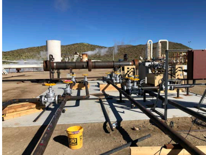
Figure 3: Equipment Pad and Partial Installation
