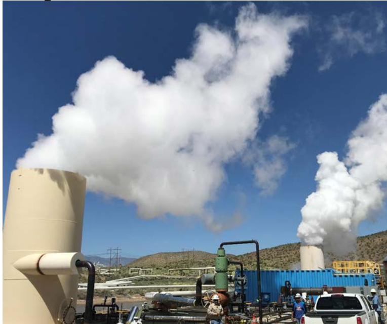
Figure 5: Installation at Well 34-A20 at Coso
