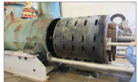
RMS manufactured Tool at work extracting Dresser Rand bundle
