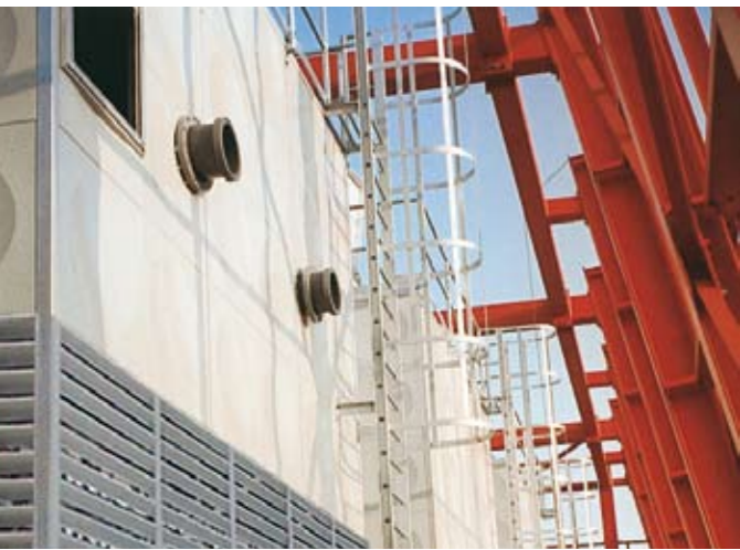
Construction and startup of a CMC Cooling tower
