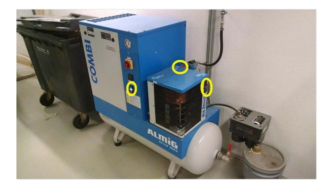
Remember to turn the compressor on before you start your job. 3 steps: start it with the green button on front, turn on cooling with the green switch on the side, and turn the red valve to let out the compressed air.
