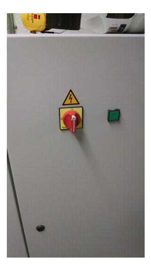
This grey box is the NC controller. Let's start by turning the red switch to the ON position, then press the green button. You should hear a light thump sound that confirms the machine is on.
