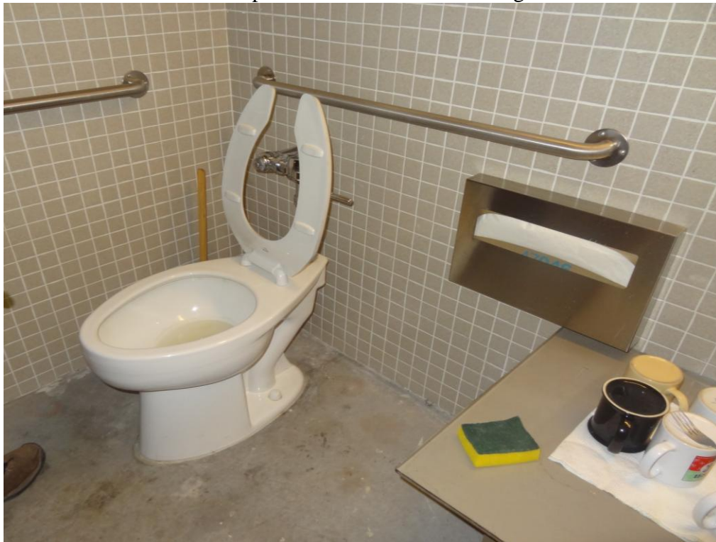
Warehouse / Shop – FCA Building #1989 Description: Restroom.
