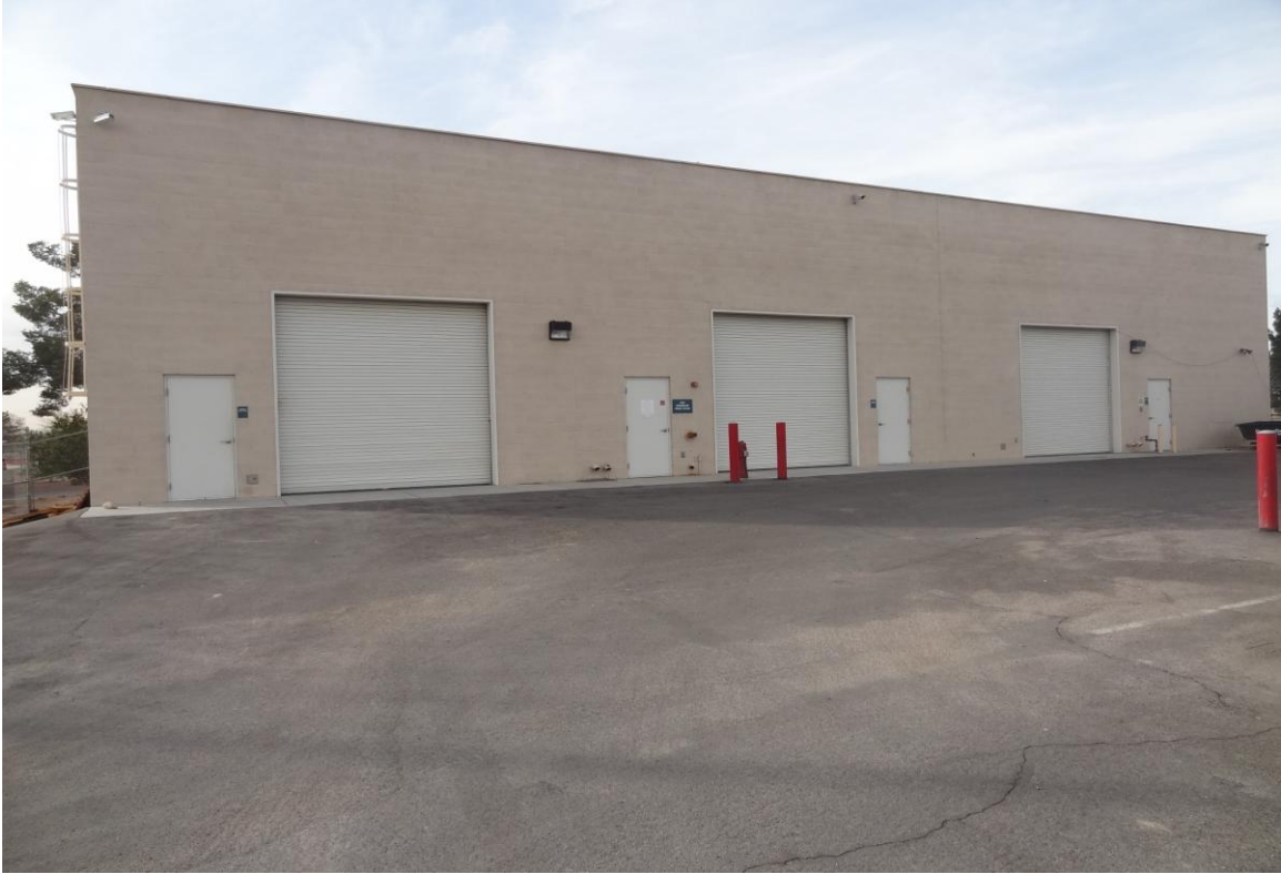
Warehouse / Shop – FCA Building #1989 Description: Exterior of the building.
