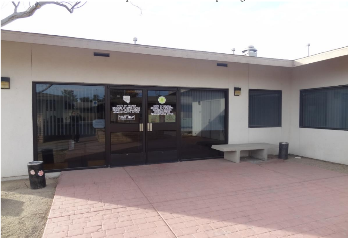
NDF / State Parks Office Building – FCA Building #2033 Description: Exterior of the building / public entrance.
