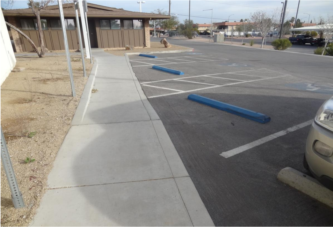
CNR / Wildlife Offices Las Vegas Site – FCA Site #9878 Description: ADA accessible parking.
