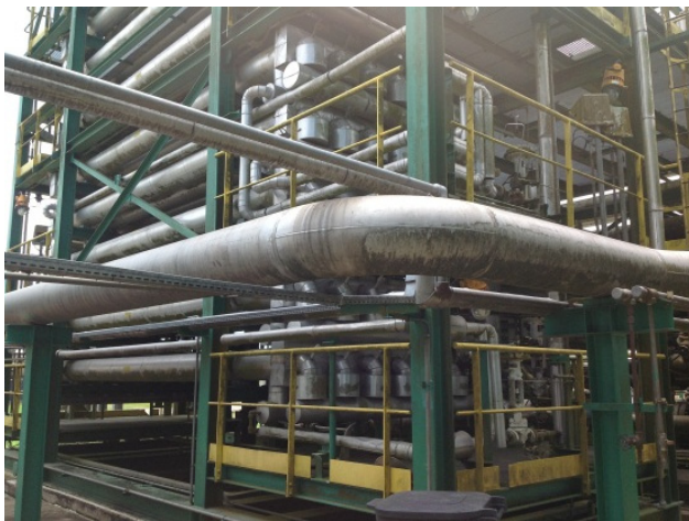
Fig. 3—Cellulose acetate membrane plant that uses the spiral-wound configuration.
