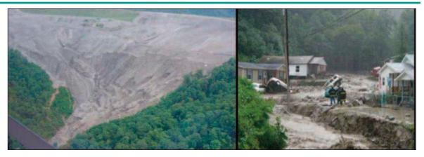
Figure 19 Lyburn flood (left) erosion and sloughing on the outslope of the durable rock fill following a storm event; (right) property damage downhill of the fill (Michael and others, 2009)
