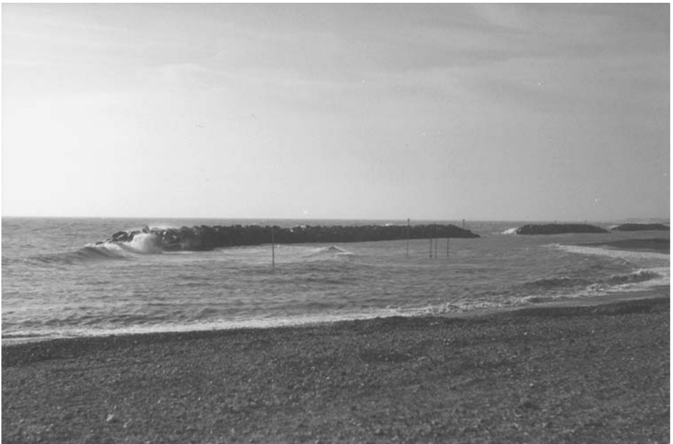
Figure 2.14(b) Photograph of real diffraction at the Elmer breakwater scheme, Sussex, England.
