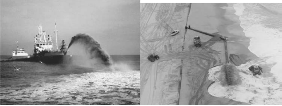
Figure 9.27 Pumped delivery of beach nourishment.
