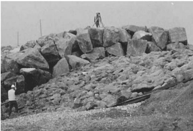
Figure 9.42 Primary armour and underlayer under construction.
