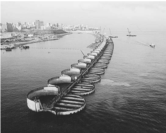
Figure 9.20 Caisson breakwater under construction.
