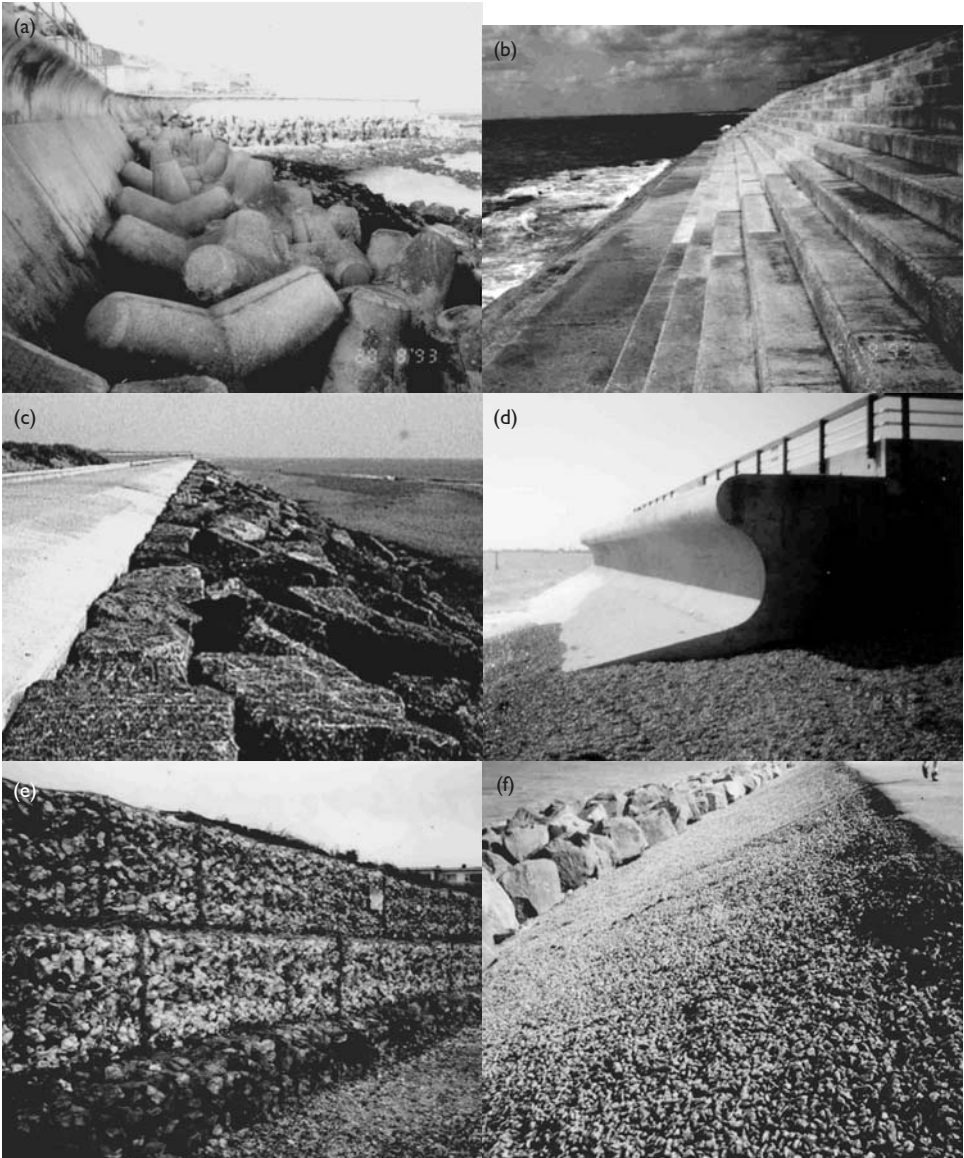
Figure 9.23 Examples of sea wall types (a) tetrapod toe; (b) stepped; (c) rock toe; (d) recurved wall; (e) Gabions; (f) open stone asphalt with rock toe.
