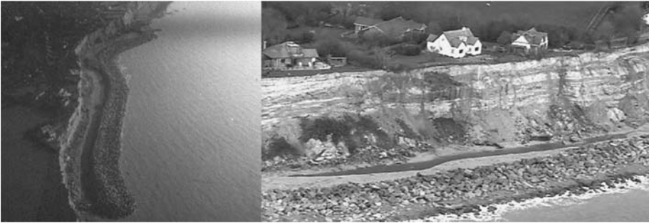
Figure 9.26 Fairlight Cove linear bund.
