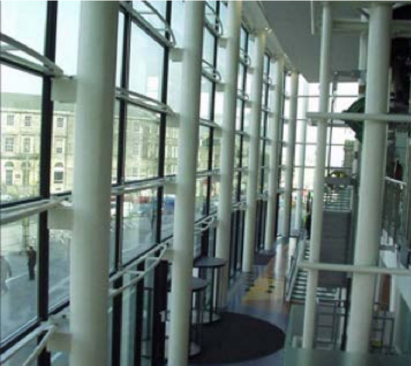
Completed installation of circular hollow structural columns
