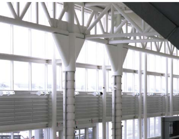
Acrylic intumescent coatings are commonly used for interior structural-steel applications.
