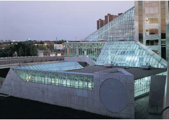
Transit station in Boston, where an intumescent fire-protective coating was applied to the structural steel.
