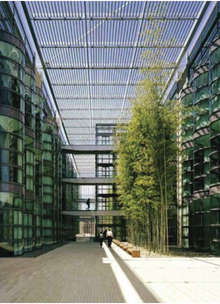
Stanford University Center for Clinical Science Research in Stanford, CA. The architectural metal was finished in a 70% Kynar 500 paint.
