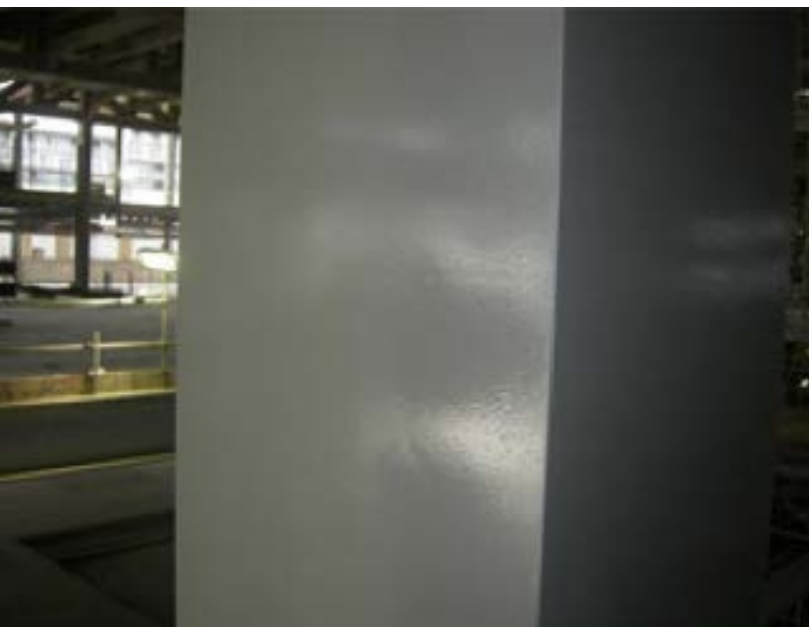
Completed installation of square hollow steel column
