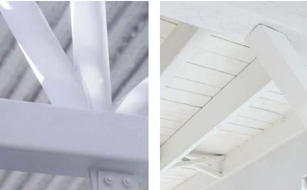
Intumescent coatings are widely used on exposed structural-steel elements, above left, but also are applied to wood substrates such as the beams and deck shown above right.
