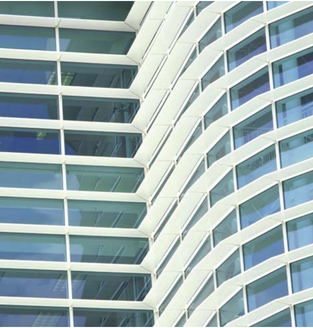
Grand Valley State University's Cook-Devos Center for Health Sciences in Grand Rapids, MI. The architectural metal was finished in a two-coat, 70% Kynar 500® paint. Photo by Wes Thompson, courtesy of Wausau Window and Wall Systems.
