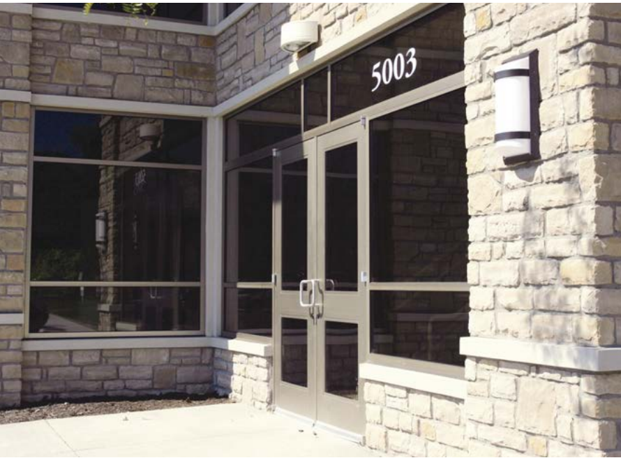
In building construction applications, anodized aluminum can be found throughout a structure's framing, in windows, doors, skylights, curtain walls, and entrances. Photo courtesy of Tubelite Inc.
