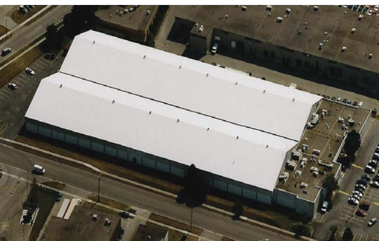
A roof-restoration coating system that includes a solar-reflective finish coat was applied to the metal roofs of the Mayfair Tennis & Racquet Clubs, Markham, Ontario. Top photo shows the coating application under way; the job is complete in photo above. The coating system—the ASTEC Metal Roof System—includes metal primer, acrylic waterproof membrane for seams and fasteners, and a white, solar-reflective, acrylic finish coat. Photos courtesy of ASTEC Re-Ply Roof Systems.
