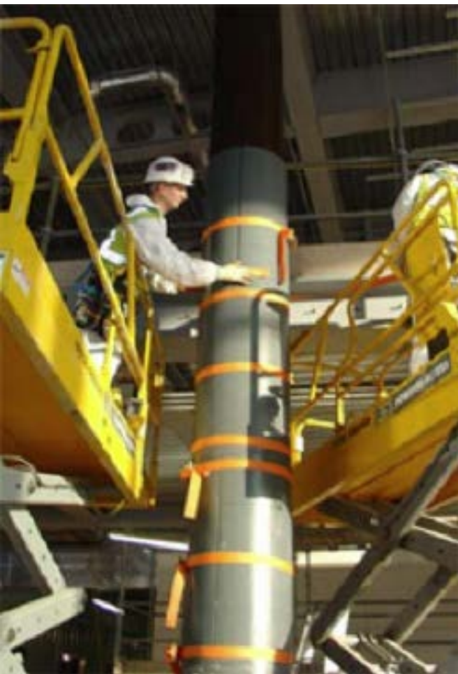
Installation of pre-manufactured epoxy intumescent fire protection
