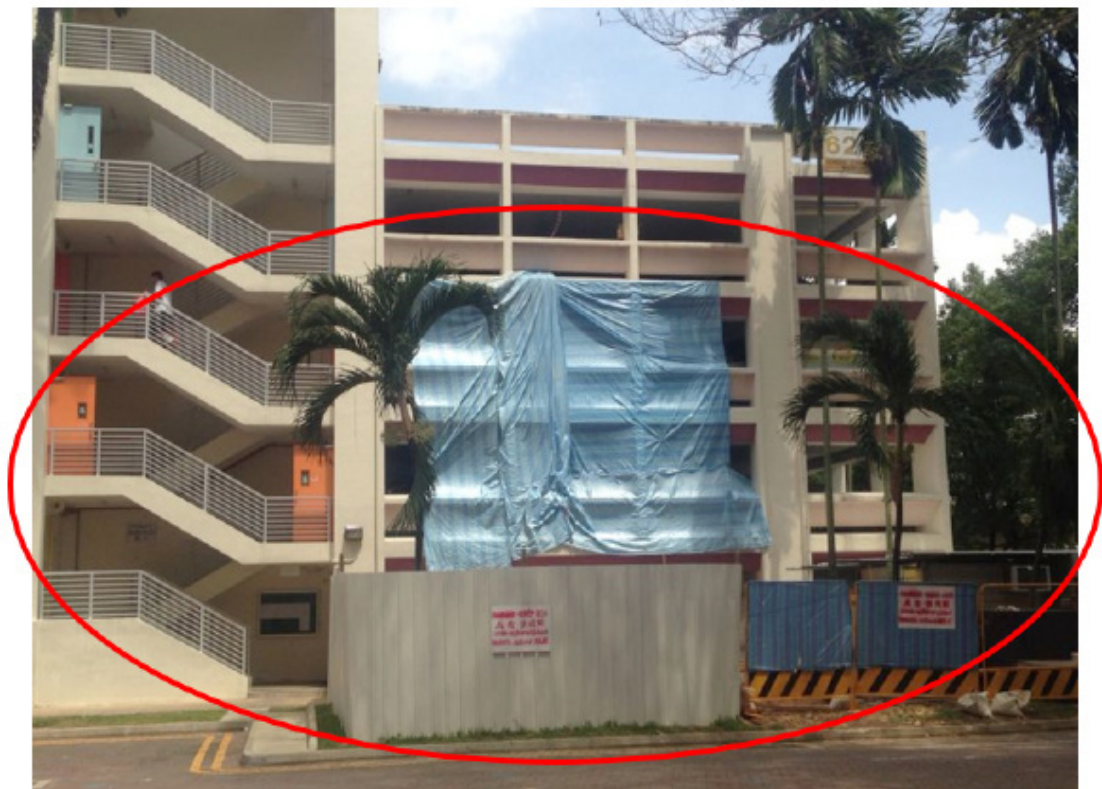
Diagram 9.9.4b.(2) - 4 : Hoarding obstructing openings for smoke dispersal
