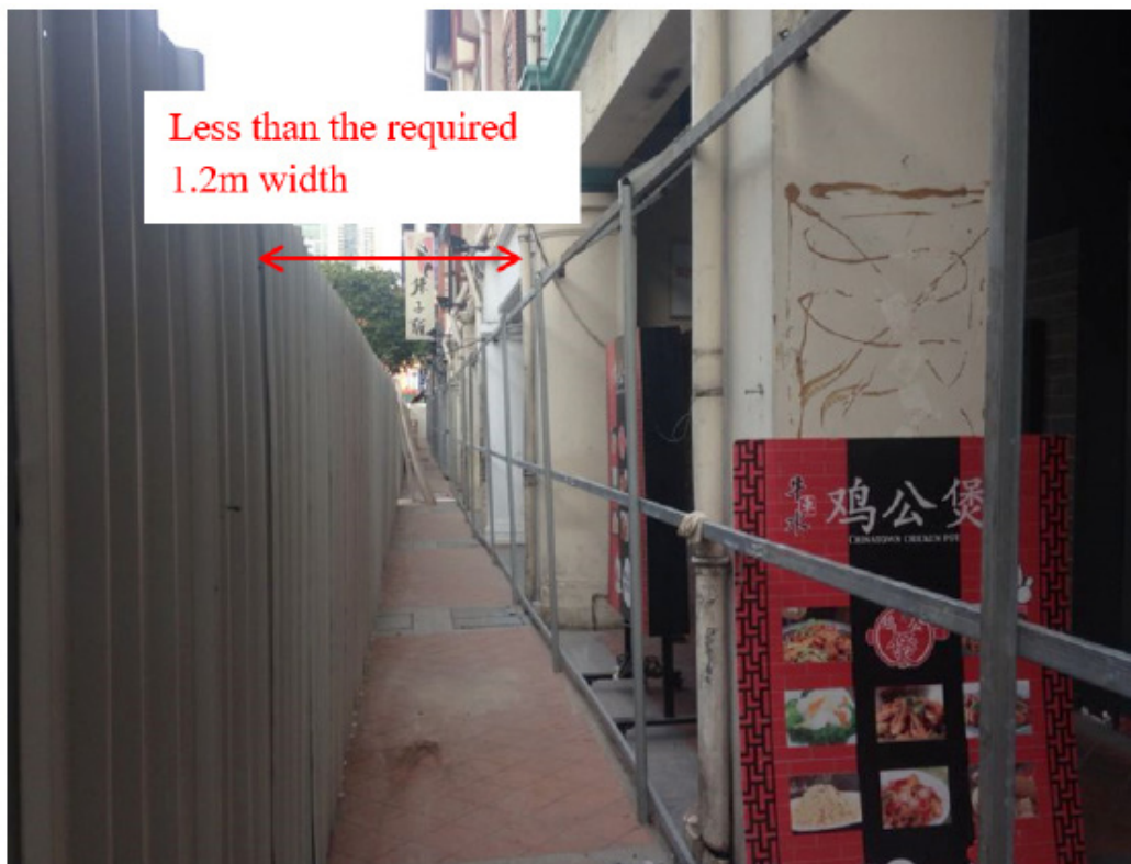
Diagram 9.9.4b.(2) - 2 : Hoarding obstructing means of escape
