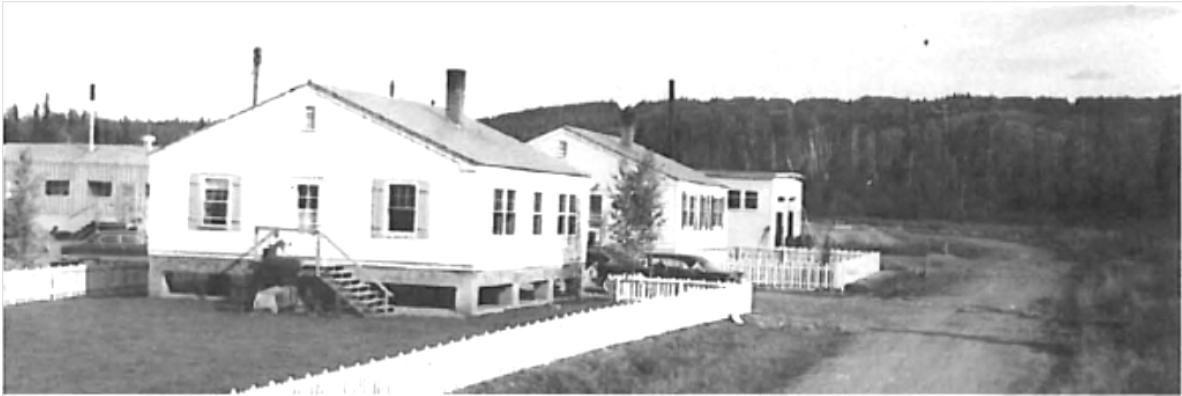
Figure 5-2: Photo of test buildings in Area 3, showing purpose-built facilities that also served as housing for researchers. 93
