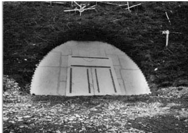
Figure 5-3: Historic image showing the original tunnel portal, circa 1969. 100
