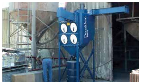
DFO - Concrete Roof Manufacturer 3,000 cfm (5,096 m 3 /h)
