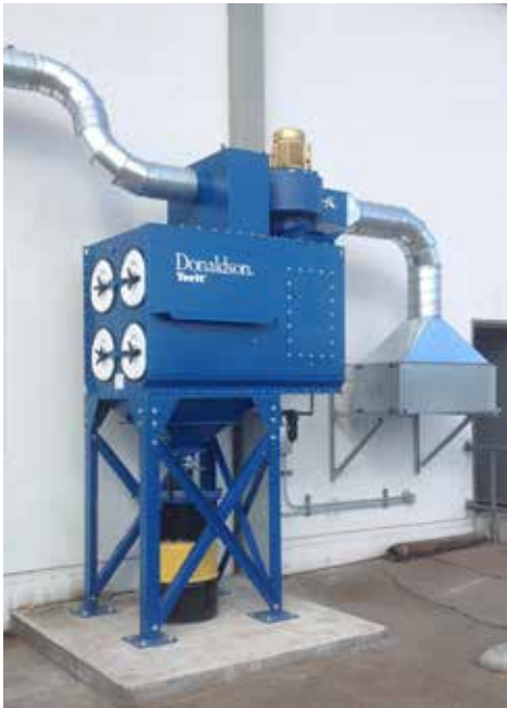
DFE on Rubber Hose Cutting 2,800 cfm (4,757 m 3 /h)
