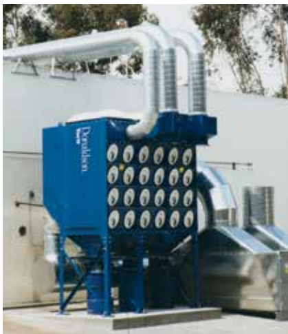
DFO on Metal Grinding 31,000 cfm (52,658 m 3 /h)
