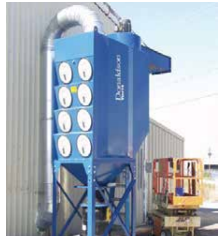
DFO on Plasma Cutting 5,000 cfm (8,493 m 3 /h)
