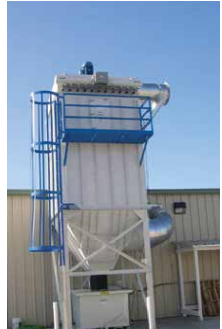
FS on Woodworking 20,000 cfm (33,973 m 3 /h)
