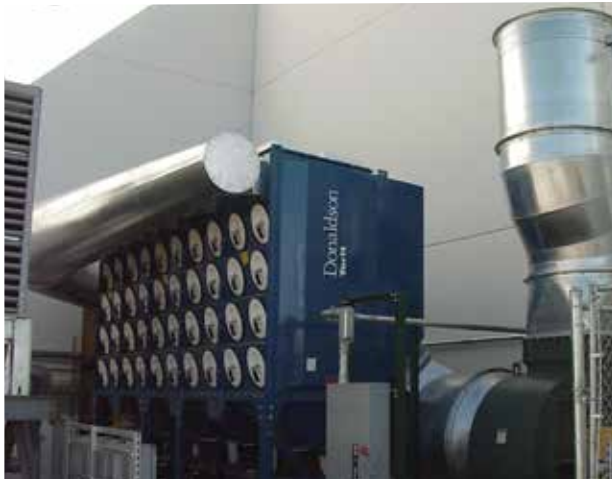
DWS ON Custom Hand Grinding 38,500 cfm (65,398 m 3 /h)
