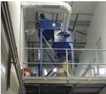
CPC on Milk Powder 1,200 cfm (2,038 m 3 /h)
