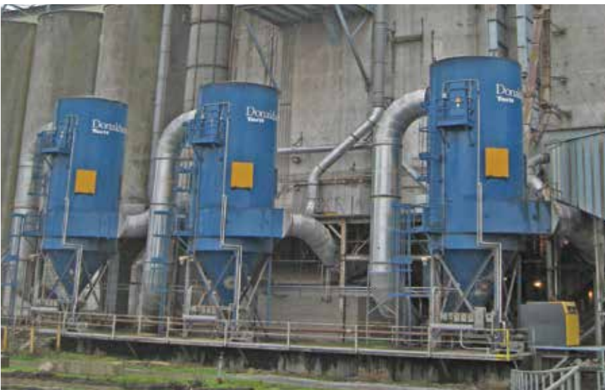
RF - Grain Terminal 61,000 cfm (103,618 m 3 /h)
