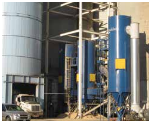
RF - Grain Terminal 34,000 cfm (57,754 m 3 /h)
