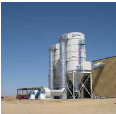
LP on Nut Dust 280,000 cfm (475,622 m 3 /h)
