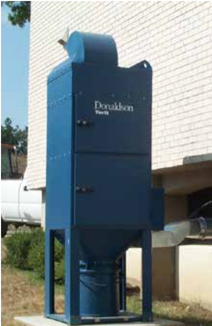
UMA - School Wood Shop 2,000 cfm (3,397 m 3 /h)
