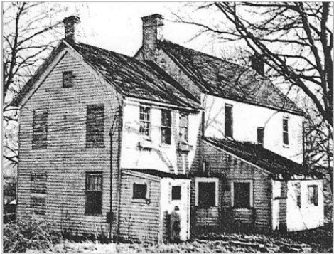
Miller's House with Millard additions. Photo courtesy of Fairfax County Public
