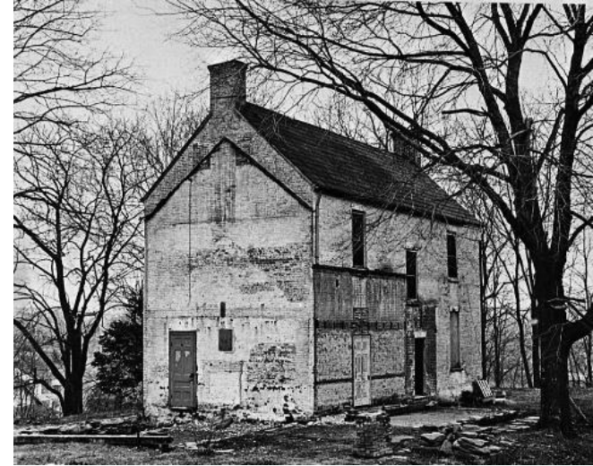
Miller's House during 1970s site restoration. Photo courtesy of Fairfax County Public Library
