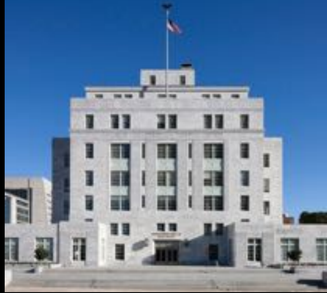
US Post Office Annex (MLK Federal Bldg) - Atlanta 1931-32
