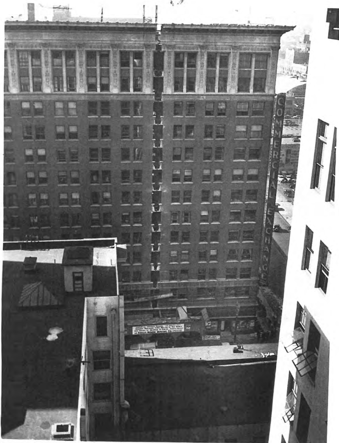
Image 8 - The building was cut in the 4 th bay. This image shows the building as relocated, prior to replacing the window sash and restoring the brick wall so the building could be reconnected. The joint is now virtually seamless and invisible. 1935 image
