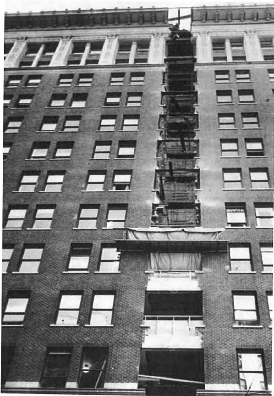
Image 7 - Relocation in progress, 1935. As a result of the move, this bay was made narrower, removing one of the windows. After the move, this bay has one window, but the change in appearance is very subtle. Photo in 1935.
