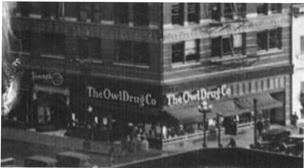
Image 3 Owl Drug Company, at corner of 8 th Street and Broadway, prior to 1935. Note also storefront on 8 th Street that is a ca. 1929 alteration. This storefront has also been retained and incorporated into the restoration of the 1924 Walker and Eisen design.
