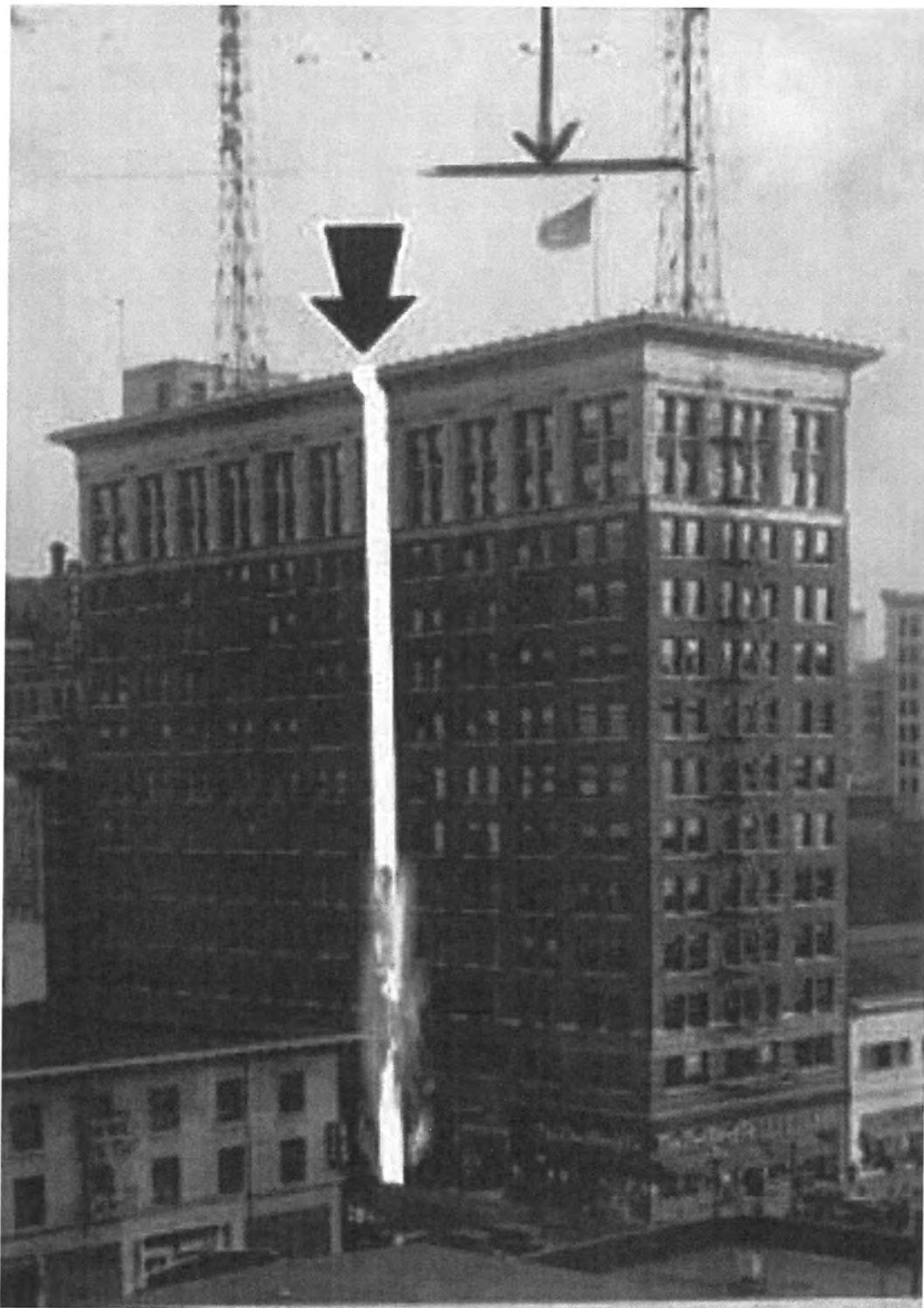
Image 6 - Cut line of building, as illustrated prior to moving. The final cut was one bay west.
