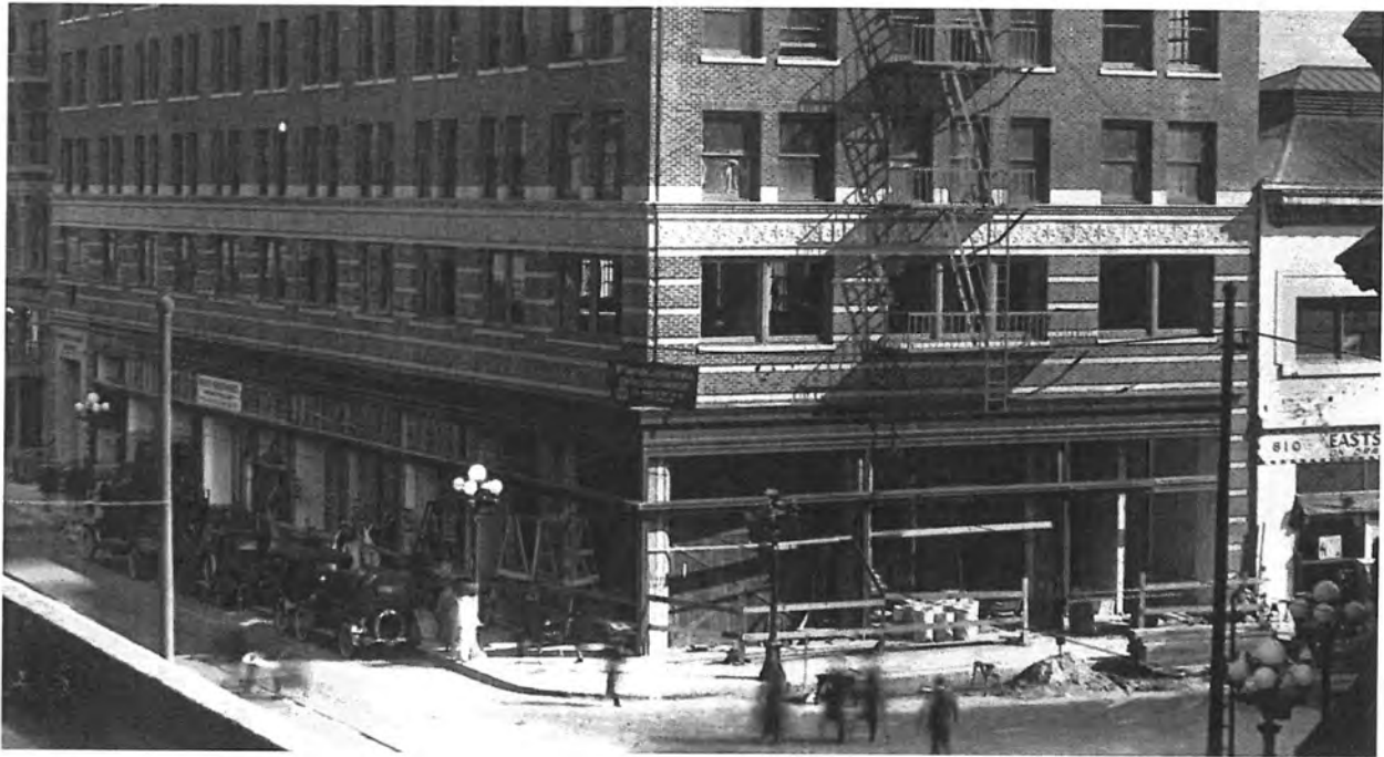
Image 2 Storefront in Progress, 1924. Note primary entrance to the building at the far left, (NE corner)
